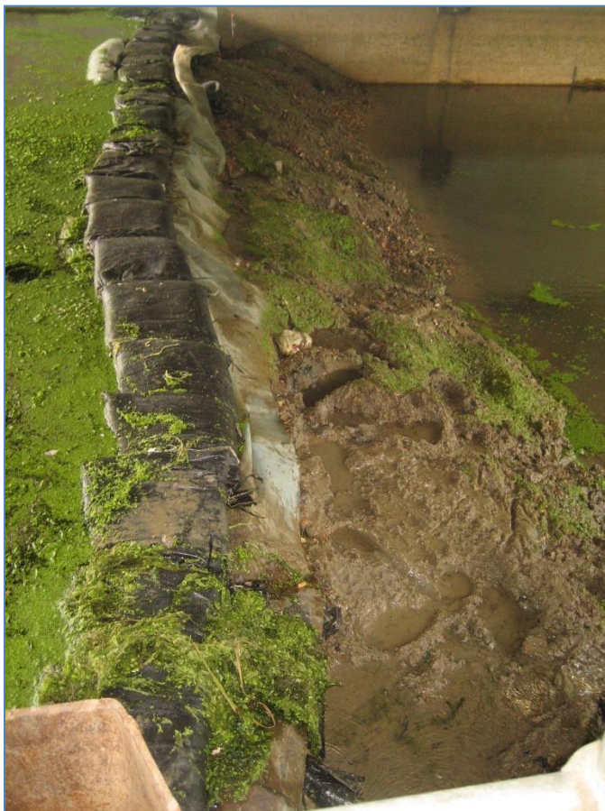
Bund constructed to prevent water backing into Moor Cut from the Green Lane Pool.
